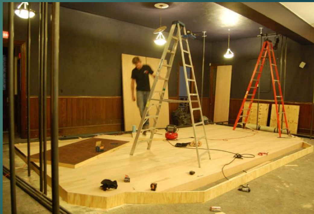
Azuka Theatre's blackbox construction inside First Baptist Church's former prayer room. Photo credit: PSP Staff.
